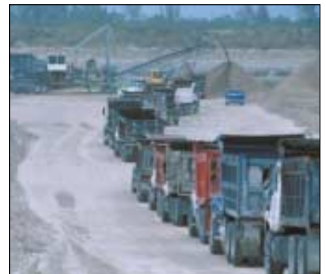
Careful mining of aggregates provides excavation of deep in-ground water storage tanks.
